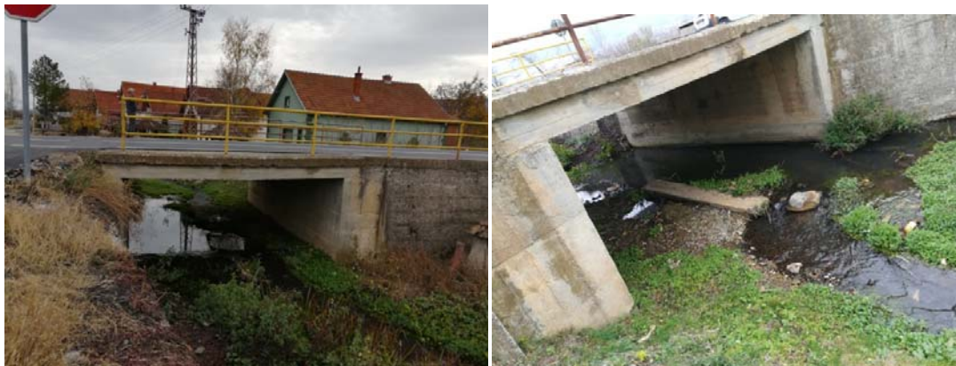
Picture 8 and 9. Intersection with Balvan stream
