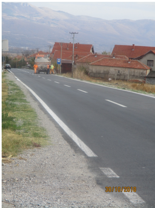
Picture 6. Part of the section with new road construction
