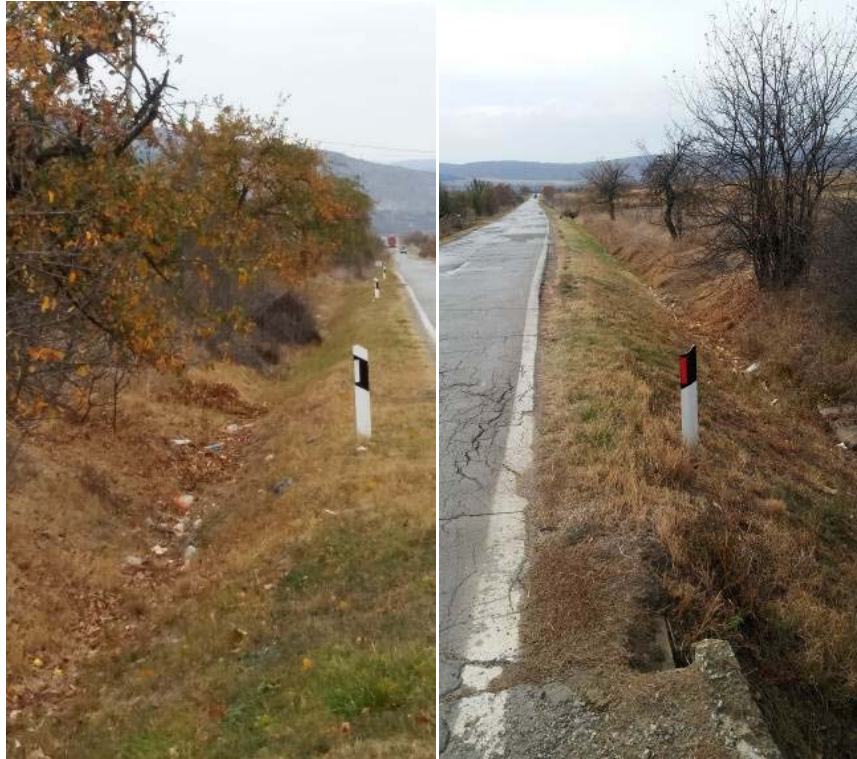
Pictures 11 and 12. Ditches along the road
