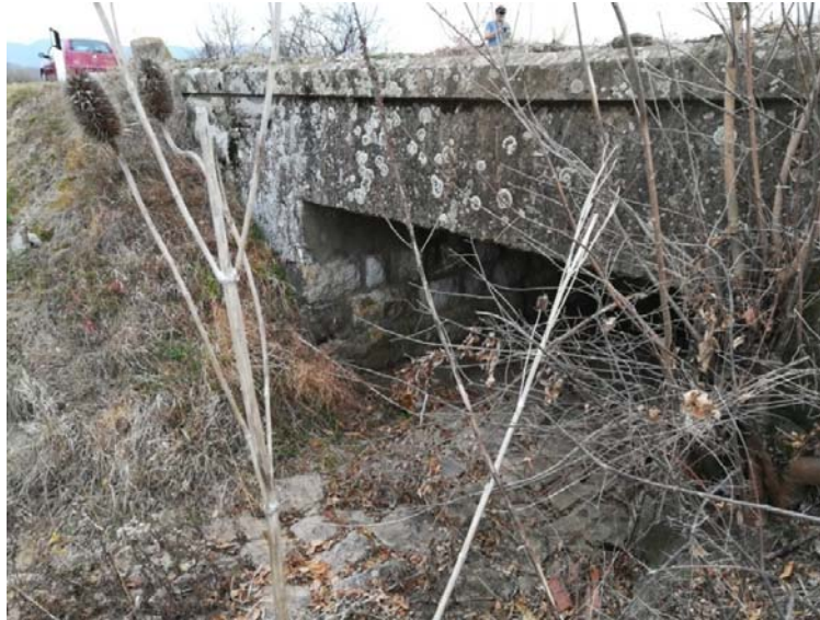
Picture 10. Intersection with occasional watercourse
