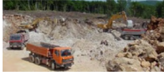
Loading of blasted material with hydraulic excavators.
