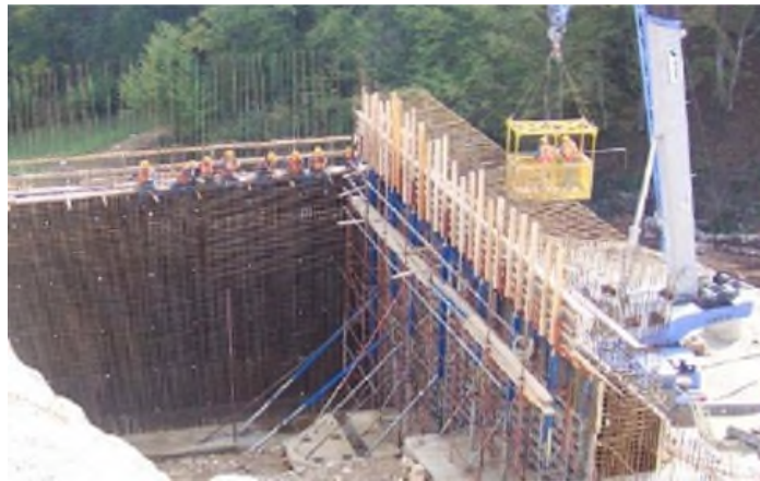
Figure 3-53. Abutment Wall Ready for Concreting.
