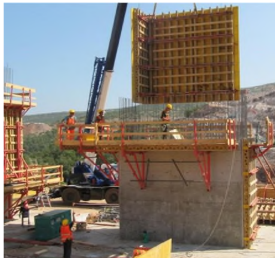
Figure 3-54. Pier Concreting
