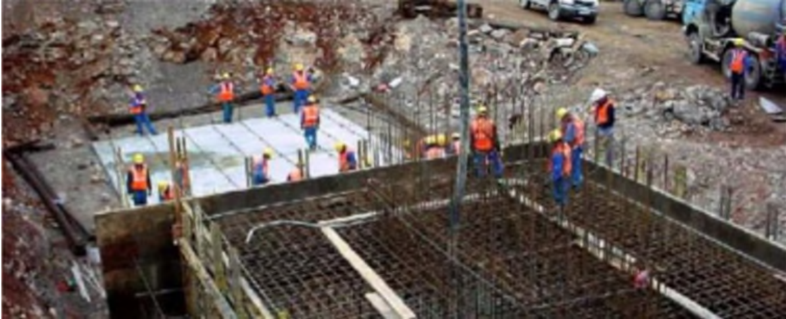
Figure 3-52. Foundation Concreting Operation
