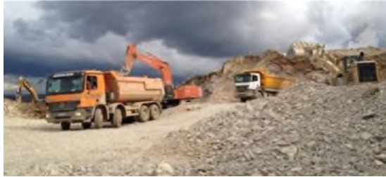
Loading of blasted material.
