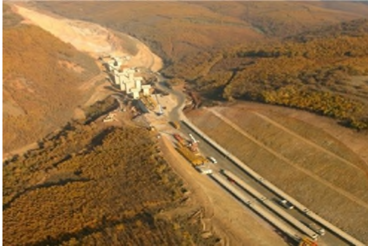
Figure 3-56. Preparation of Beam Installation
