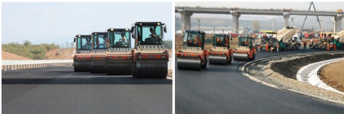
Figure 3-60. Drumrollers Compact the Asphalt Layer
