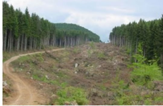
Example of area to be cleared and grubbed. (not from this project)
