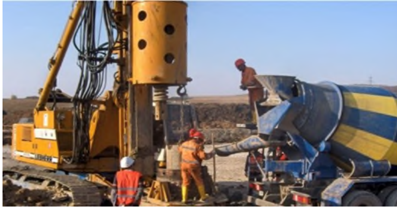
Figure 3-50. Pile Casting
