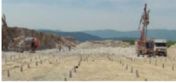
Location ready for filling with explosives.
