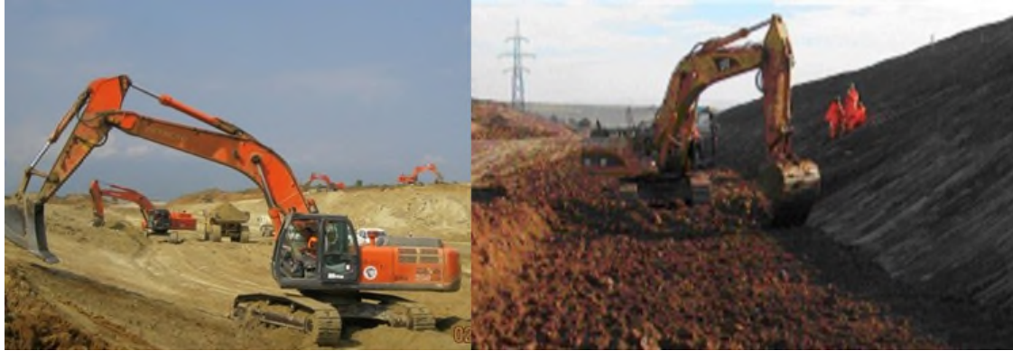
Excavation of common material with excavator.
