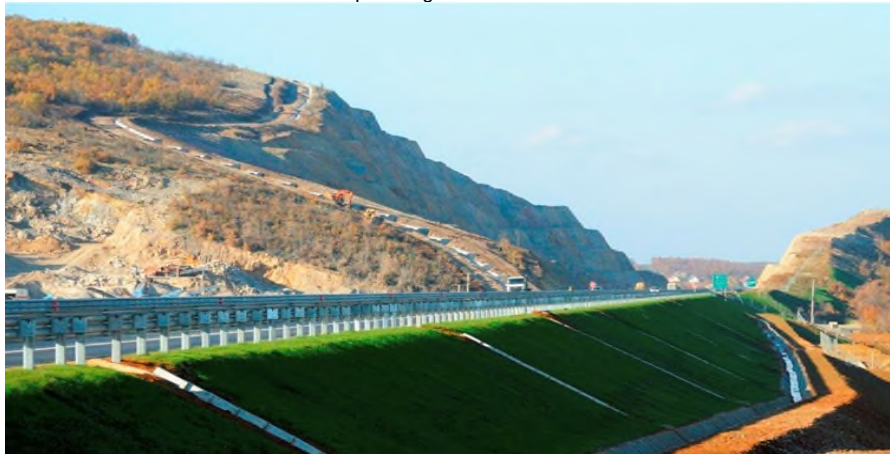
Concrete ditches and down chute construction.
