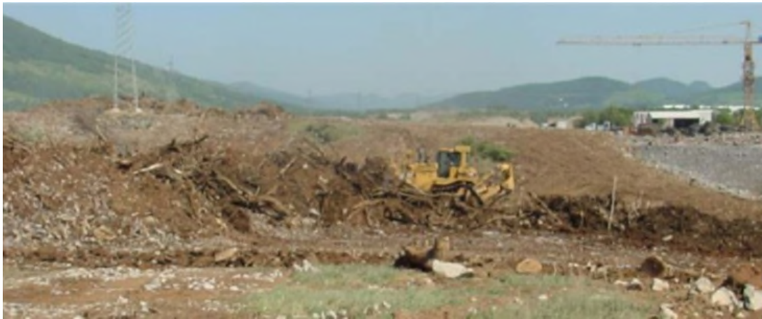
Stockpiling the cleared and grubbed material at disposal area.
