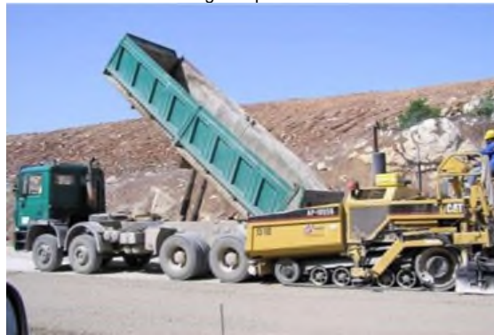
Spreading the sub-base.
