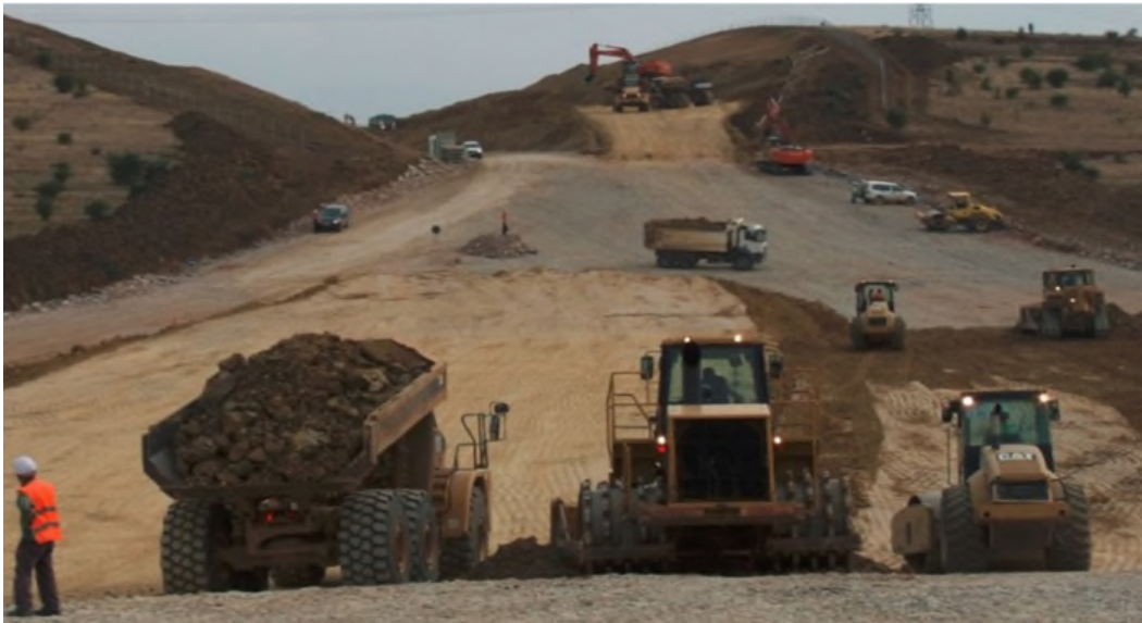
Figure 3-49. Spreading and Compaction of Gravel and Earth Materials
