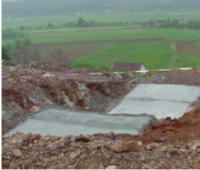
Figure 3-51. Lean Concrete Placement for Stepped Structural Foundation
