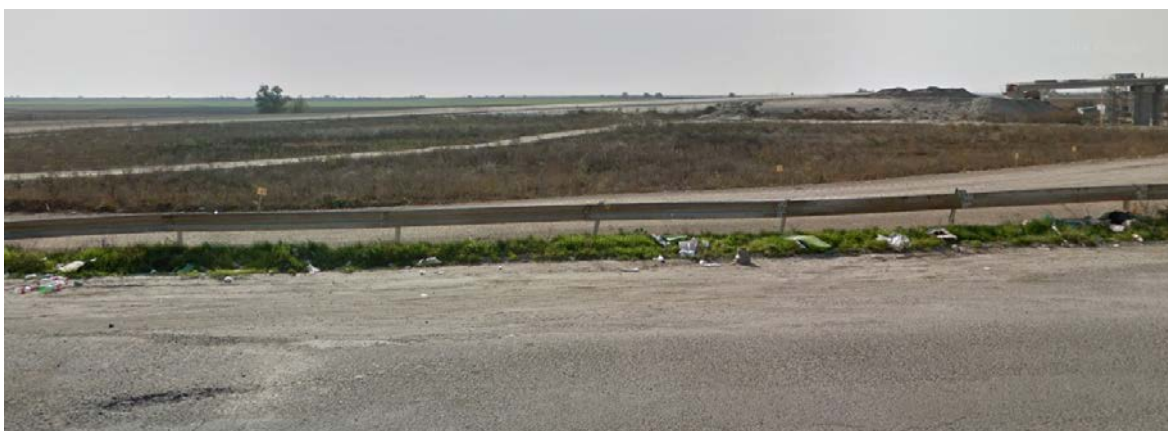
Figure No. 3: The part of the terrain for the completion of the Interchange Batajnica
